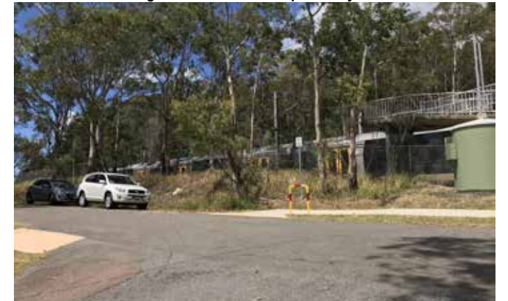
Booragul Railway Station
